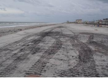
Figure 3b taken October 16, 2019 is a view from the beach berm crest looking south showing that the beach has retained most of the sand placed last year by the USACE.
