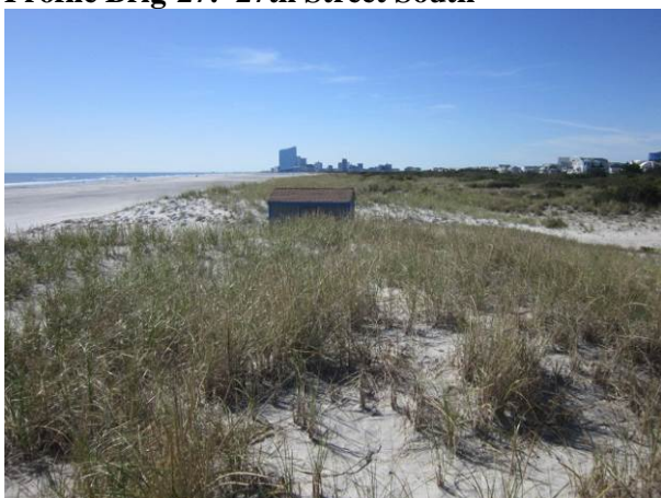
Figure 7a Photo taken October 15, 2020 presents the same perspective as 2019 with a dune system most NJ shore towns would envy. The beach remains of significant width.
