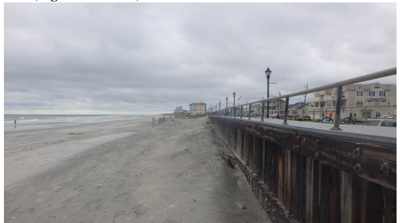
Figure 3b taken October 6, 2021 shows an additional 3 feet of vertical bulkhead indicating beach loss. The dune fencing is gone from the site path but remains in place further south. The beach is actually a bit wider with a gentler slope offshore.
