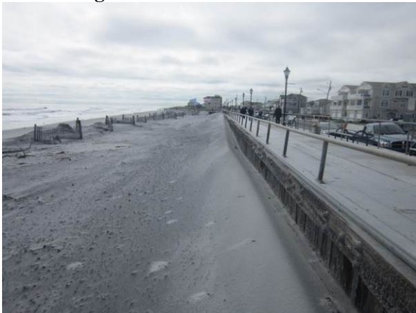
Figure 3a taken October 16, 2013, 2020 with the sand fence at the swash limit and only about 25 feet of berm left to the promenade wall. The rocks remained buried.
