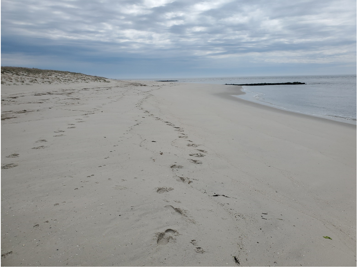
Figure 7. This view was taken April 7, 2020 at the berm crest on the beach looking east toward the rock groin. The dune toe defines the extent of dune growth leaving a modest dry beach widening toward the groin.
