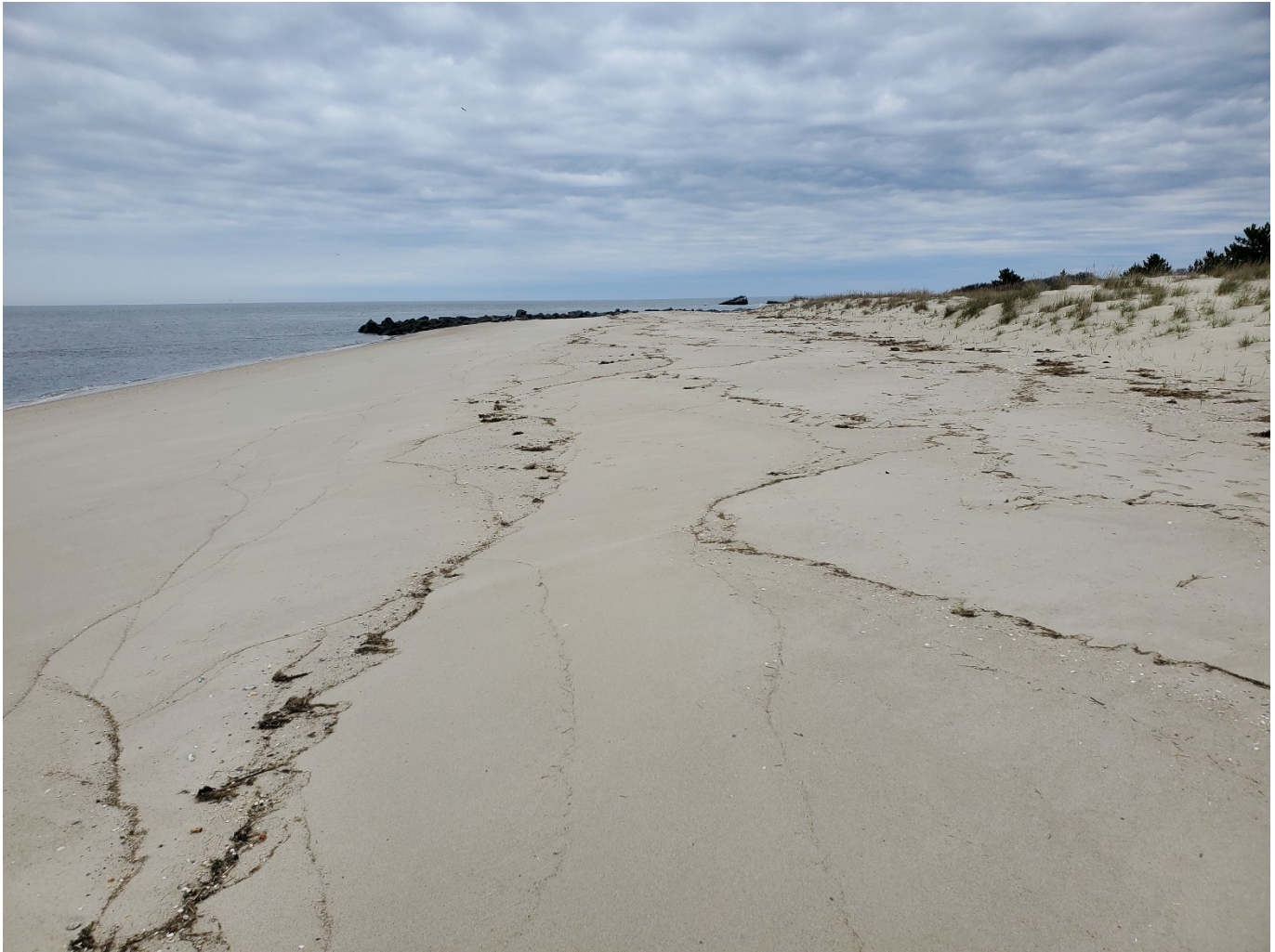
Figure 9. This westernmost cell ends at the groin in the distance. Lower Township is immediately adjacent to the structure. The wave swash has recently reached the expanding dune toe slope without causing erosion to date. The ancient concrete ship is visible in the far distance off Sunset Boulevard beach in the Township.
