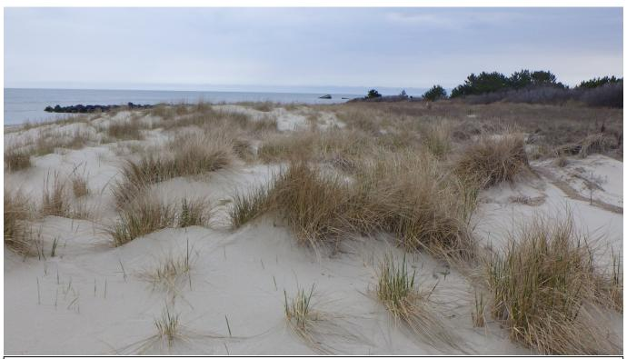
Figure 18. This westernmost cell ends at the groin in the distance. The view toward Delaware Bay was taken April 9, 2021. Lower Township is immediately adjacent to the structure. The hummocky dunes in the foreground all have appeared in the past 5-6 years as this beach has expanded.
