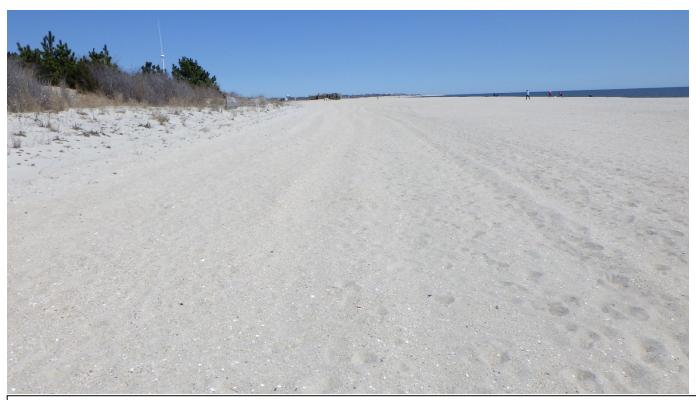
Figure 4. This view is to the northeast showing the beach width present as of April 8, 2021. The dune to the left side sits on top of the stone revetment and the beach is many times the pre-beach nourishment width creating an excellent storm barrier as well as a recreational resource enjoyed by the Borough citizens.
