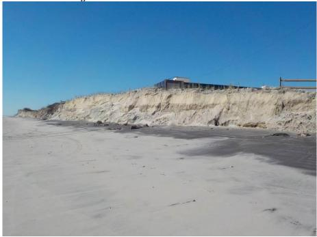
Figure 8. View from 4<sup>th</sup> Avenue looking south on October 19, 2017. The primary dune is cut back to its crest and the scarp extends south of 6<sup>th</sup> Avenue. No dry beach remains, so waves reach the dune each high tide.
