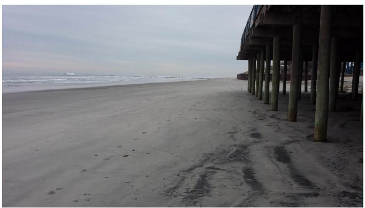
Figure 20. A close up view of the beach at the very seaward end of the timber pier indicating that no dry beach or dune feature remains at the pier's end (March 2017). Visible between the pier pilings is the repositioned dune between this pier and Morey's Surfside Pier.
