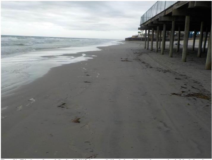
Figure 21. This view to the south October 27, 2017 shows nearly identical conditions at the seaward end of the timber pier between 23<sup>rd</sup> and 24<sup>th</sup> Avenues. Waves readily reach under the pier on a very flat beach. The revised dune system shows in the distance beside Morey's Surfside Pier so beach width is critical to this site's ability to moderate wave action.
