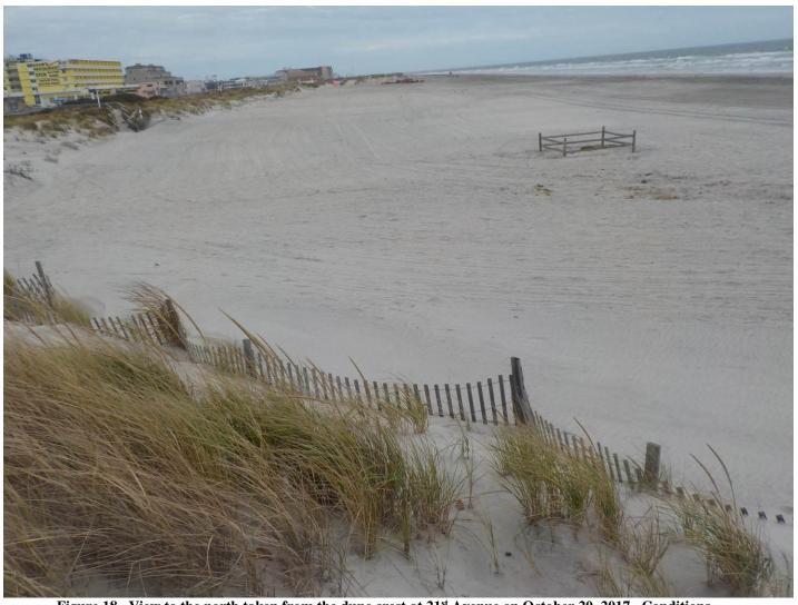
Figure 18. View to the north taken from the dune crest at 21<sup>st</sup> Avenue on October 20, 2017. Conditions remain stable at this site with wind-transported sand having nearly buried the dune fencing along this section of the oceanfront beach.
