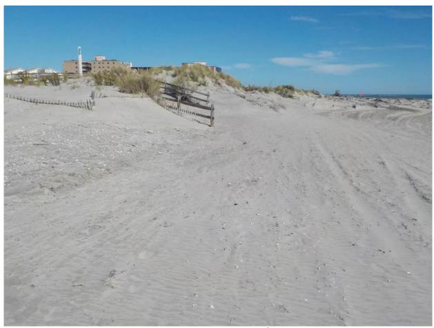
Figure 12. View to the north taken from the toe of the dunes at 11<sup>th</sup> Ave. October 19, 2017 following spring sand placement and some accretion at the repaired scarp.
