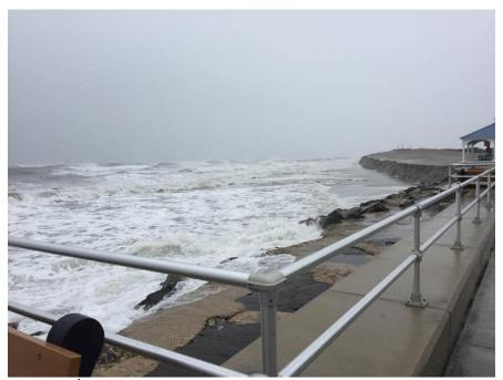
Figure 7. View from the 3<sup>rd</sup> Avenue gazebo looking south taken during the March 14, 2017 northeast storm. A significant scarp in the seaward dune is shown along with observed recreational beach elevation and shoreline losses and waves breaking on the revetment.
