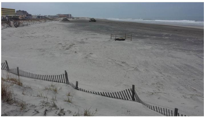
Figure 17. View to the north taken from the dune crest at 21<sup>st</sup> Avenue on March 23, 2017. Sand continued to accumulate at the dune fencing installed after Hurricane Sandy and work in the distance was underway to recover sand from the beach berm to use on pedestrian beach access paths and at the dune toe where needed.
