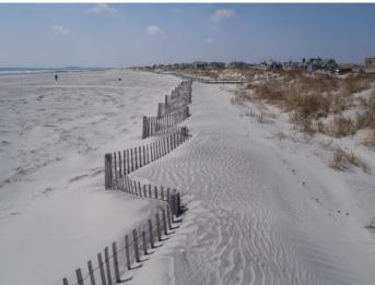
Photoplate 7b – Photo taken April 10, 2018 showing continued sand deposition around the fencing.
