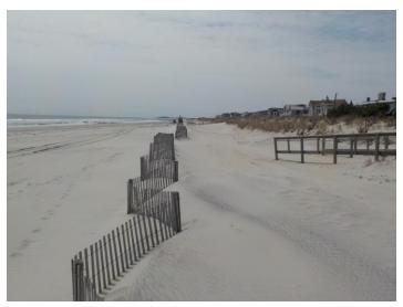
Photoplate 4b - Photo taken April 9, 2018 shows the winter's accumulation of sand around the new fence. This beach changed very little during the year.
