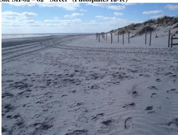
Photo 1a – Photo taken October 3, 2017, this was the fall after the beach restoration where dune fence posts had been installed for a new dune toe fence.
