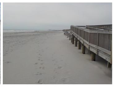
Photo 3b – The April 9, 2018 photo shows the entrance ramp positioned at the dune toe alignment with a dry beach seaward.
