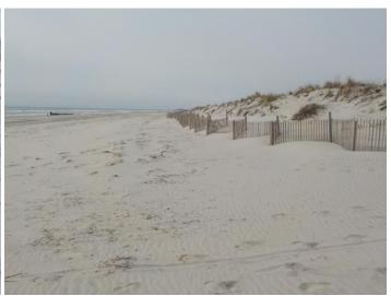
Photo 1b - Photo taken April 9, 2018 following a series of mild to moderate northeast storms, no damage was seen at the dunes where the fencing installed is a third buried.
