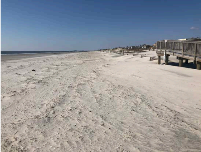
Photo 3a - The April 16, 2020 photo presents a wider dry beach with sand added to the nearly buried sand fencing at the toe of the seaward dune slope.
