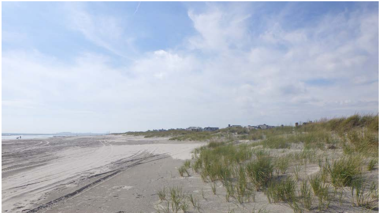
Photoplate 7c – Photo taken October 4, 2021 showing a series of steady dune grass growth and sand being added to the seaward toe.
