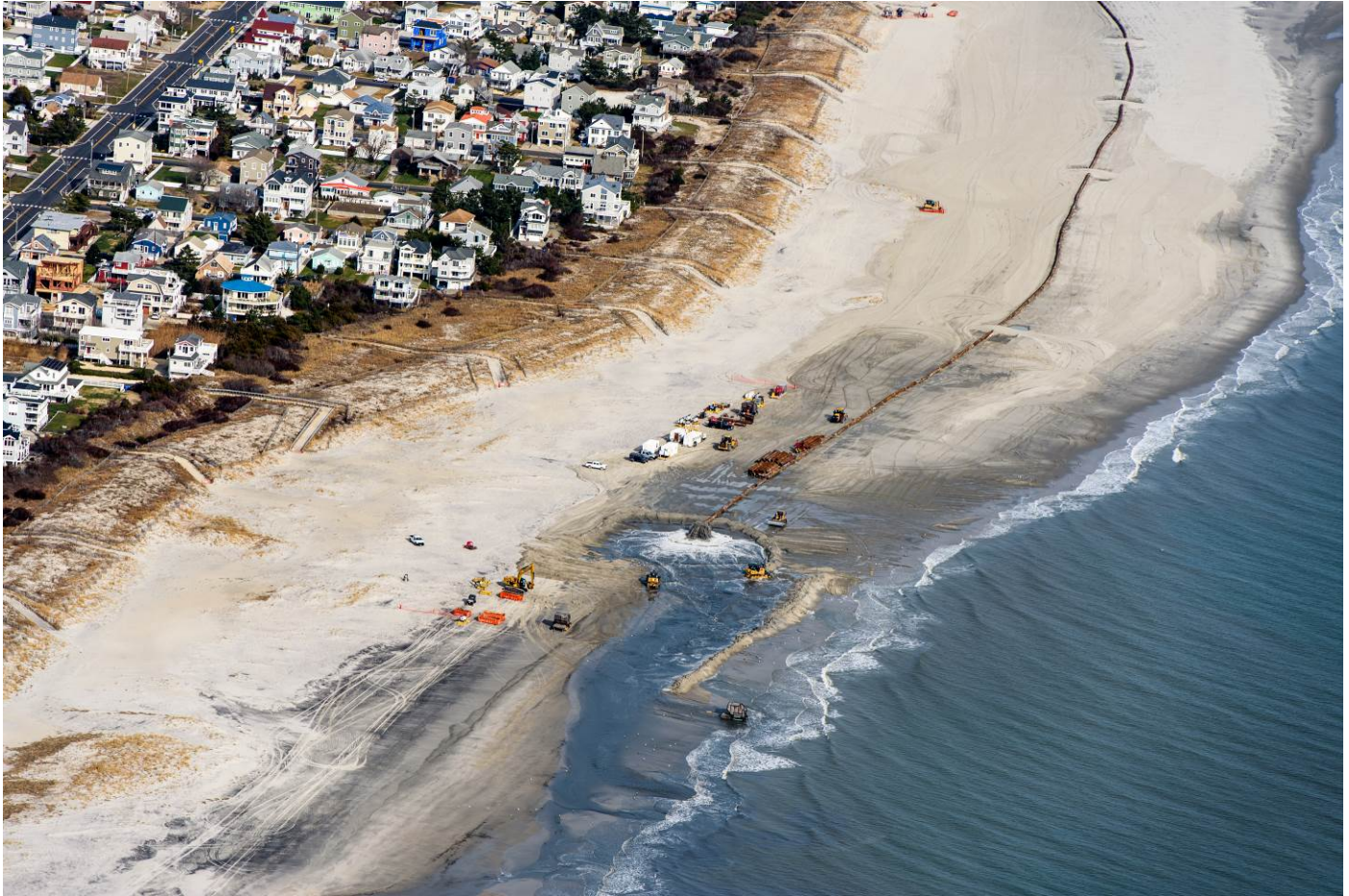
Above is an aerial view of Strathmere, taken December 7, 2019, showing the sand placement operation underway south of Tecumseh Avenue as the maintenance operation proceeded. (Photo by Ted Kingston).
