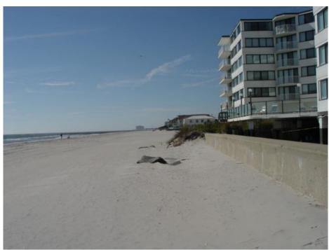
The Longport site is about 15 blocks from the terminal jetty to Great Egg Inlet at 11<sup>th</sup> Street. This October 22<sup>nd</sup> 2007 photograph shows the concrete seawall with sand ramped up to within three feet of the crest. Note that the armor stone seaward of the wall's base just barely appear. Insufficient beach width exists to establish a dune along this segment of shoreline.
