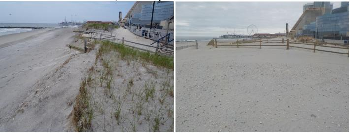
This profile site is located near the Absecon Inlet south jetty. The June 21, 2016 (left, view to the south) shows a scarp cut into the dune with damaged fence and steps remaining at the beach access path. The right photo (taken December 22, 2017) shows the restored beach and dune following the USACE 2017 maintenance project.
