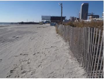
This location is also within the Absecon Island Federal shore protection project just south of Steel Pier. The left photo, taken December 22, 2017, shows the beach under construction. Photo shows the beach and seaward dune toe one-year post construction (November 21, 2018). At this location, the project beach is relatively stable and supports the established dune.
