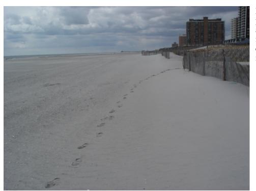
Figure 213. At Raleigh Avenue in Atlantic City the Federal beach project converted a moderate width beach with a small dune system into an expansive dry beach with a substantially larger dune system following project completion. Since 2004, the beach has remained essentially unchanged as the losses were matched by gains from the north or offshore.
