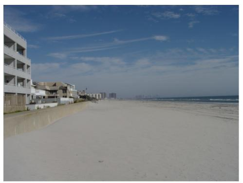
Figure 230. The October 22, 2007 photograph was taken seaward of the concrete seawall and shows the sand elevation at the wall and the width of the beach. The sand volume declined by 5.69 yds<sup>3</sup>/ft, and the shoreline retreated by 5 feet between the spring of 2006 and the fall of 2007.
