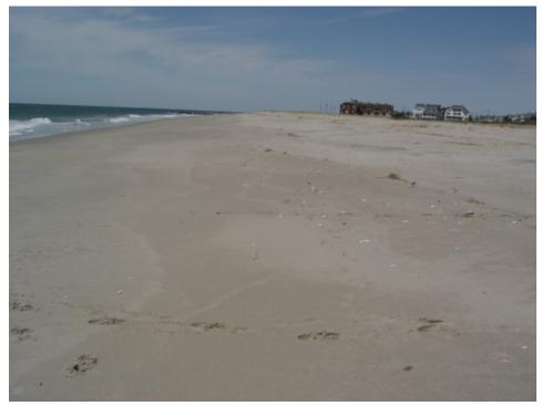
Figure 296. The vegetation is beginning to colonize the wide berm following beach restoration. High level recreational activity prevents it from growing in front of the profile site at the beach club. The sand volume increased by 16.92 yds<sup>3</sup>/ft., while the shoreline advanced 22 feet. Initially not a stable nourished beach in the early 1990's, the site has become very stable as the shoreline south was built seaward to support this width.
