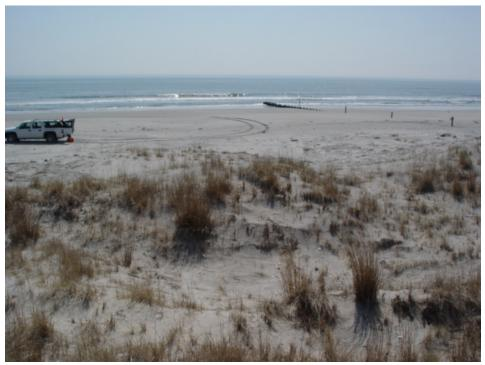
Figure 293. This view taken November 21, 2007, shows the extent of the dune system and the native vegetation across this wide area. The beach gained  $5.76 \text{ yds}^3/\text{ft.}$ , and the shoreline advanced 14 feet over the past 18 months. The dense vegetation prevents sand from reaching inland beyond the small fore dunes that are developing at their seaward limit.
