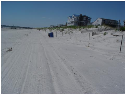
Figure 262. By November 9, 2007 the sand fencing had been replaced with a zigzag pattern in an up-slope position on the seaward dune profile. The structure in the foreground on the beach is a storm water outfall pipeline, not a groin. The Borough of Avalon is the distant skyline showing the barrier island offset at the inlet. The beach lost a minimal  $2.44 \text{ yds}^3/\text{ft}$ . with a minuscule shoreline advance of 0.27 feet.
