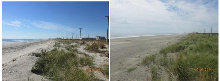
The dune here at the 1<sup>st</sup> Street location consists of a geotextile core covered by sand. Storm damage was minimal and natural recovery has blended in well with the surviving vegetation. The majority of the accumulation has been in the form of a wider beach and much larger summer berm. Sand moved onto the shoreline from bars built offshore.
