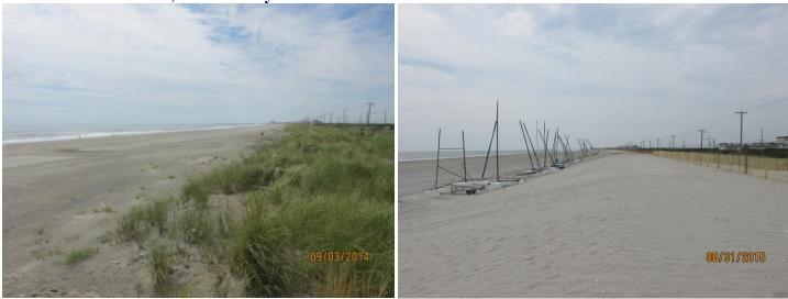
The dune here at the 1st Street location consists of a geotextile core covered by sand. Storm damage was minimal and natural recovery has blended in well with the surviving vegetation. Photo on left taken September 3, 2014 at the toe of the original dune finished in 1998. Right photo taken August 31, 2015 following the federal project building an addition to the dune plus the new beach template.
