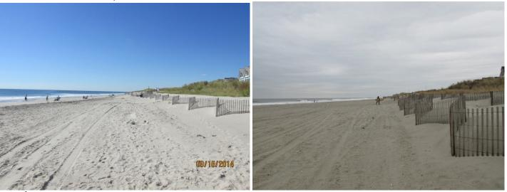
The 9<sup>th</sup> Street site is located near the Townsend's Inlet south jetty. There was no wave attack on the properties due to Sandy and the beach was restored during 2013. The dune fence shows a considerable accumulation at the fence with a narrow beach beginning to emerge to the south by September 15, 2014. The right photo taken, on October 7, 2015, followed an Avalonfunded beach restoration in 2015 augmenting the post-Sandy federal work in 2013.
