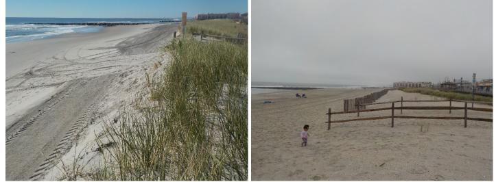
The left photo (taken October 2, 2017) shows a beach still present from the USACE (2013) beach fill, but with high tide at the eroding dune toe. The right photo (taken October 8, 2018) shows sand placed up to the scarped dune vegetation line.
