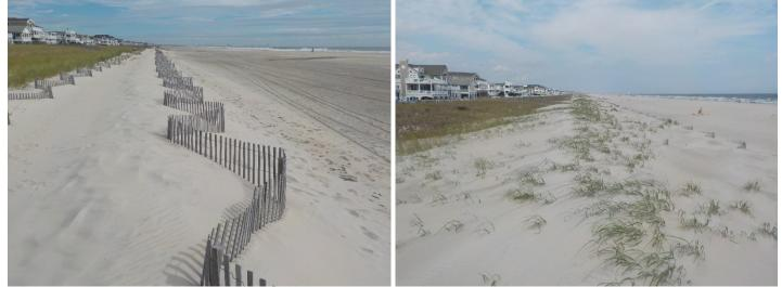
In 2015, the 56<sup>th</sup> Street site received its first sand replenishment since the 1995 state beach fill. The new dune was planted and fenced as shown on the left photograph (September 22, 2017). The right view was taken September 18, 2018 and shows that the newest line of sand fencing has been completely buried by Sept. 2018.
