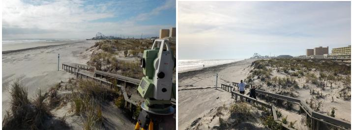
The 15<sup>th</sup> Avenue site is just south of the locus of major erosion problems in North Wildwood. The November 15, 2017 view to the left shows storm debris deposited at the toe of the dune with a dry beach pocket remaining near 20<sup>th</sup> Avenue to the south. By November 1, 2018 the situation had improved a bit with a wider beach, but note that some dune retreat had occurred (distance from the white pole to the dune slope).
