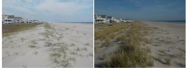
In 2015, the 56<sup>th</sup> Street site received its first sand replenishment since the 1995 state beach fill. The new dune was planted and fence that was placed is virtually covered by sand as shown on the left photograph (September 18, 2018). The right view was taken November 11, 2019 and shows that the newest line of sand fencing remains buried by accreting sand with the foredune vegetation growth remaining strong.
