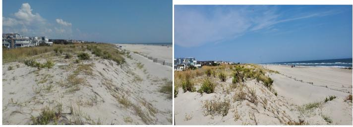
The left photo (September 6, 2018) follows the 2017 federal maintenance. The right photo taken on September 23, 2019 shows the foredune fencing virtually covered by accreting sand, while the berm elevation has eroded back minimally.
