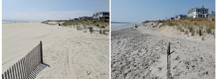
The 9<sup>th</sup> Street site is located near the Townsend's Inlet south jetty. The fall of 2018 survey (left photo taken September 10, 2018 shows the recreational beach remained usable to beach goes, though eroded back from the placement of sand following the most recent beachfill. The erosional trend of the recreational beach continued through the fall 2019, but the dune here was not affected. (Right photo taken October 15, 2019.)
