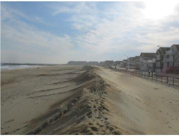
By May of 2014 the beach had 82.26 yds<sup>3</sup>/ft. in new sand added by the USACE resulting in a 113-foot shoreline advance. The Dec. 22, 2014 view on the left shows a single fence and no dune, while the Dec. 11, 2015 view on the right shows that the municipality had pushed up a sand ridge as a winter "dune". This precludes any sand building around the fence line.
