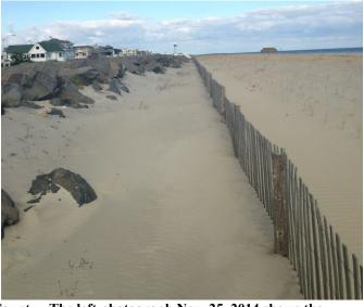
This site has the worst erosion history of any site in Monmouth County. The left photograph Nov. 25, 2014 shows the completed work by the USACE after one year following a 180-foot berm crest retreat. On the right the existing beach has narrowed further with a single straight line of snow fencing in place to start a dune on site as of Dec. 24, 2015.
