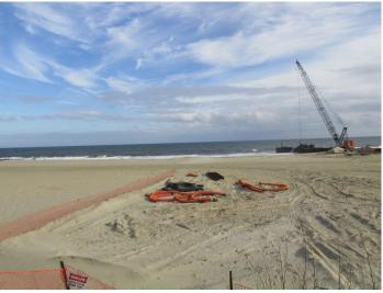
The Darlington site has a small sub-aerial beach contained between two larger groins. The upland bluff was eroded significantly during Sandy and added to the beach sand. By November 14, 2014 (left) natural recovery added 26.32 yds<sup>3</sup>/ft. back to the beach with some reconstruction of bluff protection structures. A year later (Nov. 30, 2015) the USACE project was underway adding dramatically to the beach with additional groin work in progress as well.
