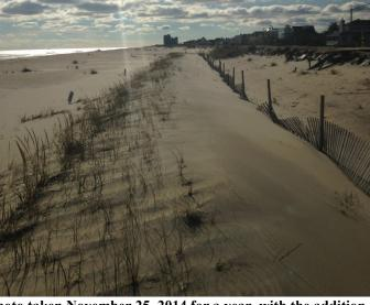
The restoration by the USACE had been completed in the left photo taken November 25, 2014 for a year, with the addition of 101.64 yds<sup>3</sup>/ft. to the profile's cross section. A small dune was added by the summer of 2014 as sand was redistributed somewhat at the water's edge and enhanced by December 24, 2015 with wind transported sand.
