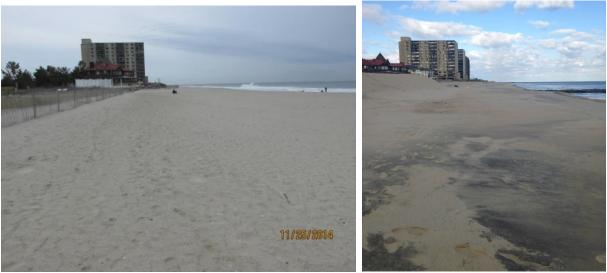
The left photo taken November 25, 2014 shows the results of the USACE work to restore the project to design specifications a year following completion. To the right the beach has narrowed exposing the groin by December 3, 2015.
