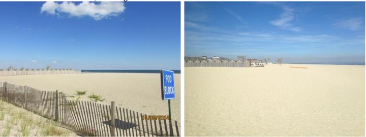
By October 8, 2014 the USACE had restored the beach width and a dune was added from sand extracted from inland and the material ramped up to the rock seawall. The dune developed and by Sept. 16, 2015 was well vegetated with a wide, dry sand beach seaward shown by the view to the north including the fencing that defines the property line.
