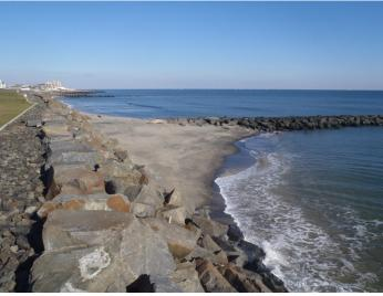
This profile is located between two rock groins that limit sediment movement. This area has never received sand from direct beach nourishment. The photo on the left (taken November 21, 2014) shows the deposit of sand derived from the storm erosion of the bluff. By December 4, 2014 sand moved offshore and adjusted lower at the rocks.
