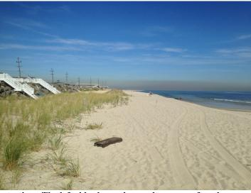
This site is near the northern limit of the initial Federal shore protection. The left side shows the results a year after the placement of 40.12 yds<sup>3</sup>/ft. of new sand and a new dune on the beach by Oct. 8, 2014, while the right side (Sept. 16, 2015) shows how well the dune grass developed and added material to the dune.
