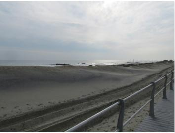
The USACE completed restoration in 2014 adding 32.29 yds<sup>3</sup>/ft. The view on December 11, 2015 shows a similar beach width with the winter storm "dune" in place seaward of the boardwalk. The vegetated dune still exists landward of the boardwalk.
