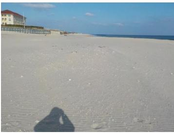
The Darlington site has maintained the as-built width quite well. Completed early during Phase III, there is a wide beach with a berm extending 340 feet beyond the bluff. The bluff is once again protected behind new timber bulkheads.
