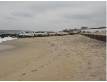
This site is located on the highest point along the bluff shoreline. The photo on the left (taken December 12, 2017) shows the new beach after some adjustment. The vertical bulkhead just shows to the right side. By December 2018 the four pilings and a rock that show on the left are part of a fully exposed groin with the bulkhead more extensively exposed as well.
