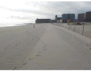
This site is the northernmost location in the Phase II part of the Monmouth County project. The left photo was taken Nov. 28, 2017 and shows the sand fence placed primarily to restrict access to the boardwalk reconstruction. Sand did accumulate at the toe of the fence as the boardwalk work continued. No storm ridge was pushed up as of mid-December 2018.
