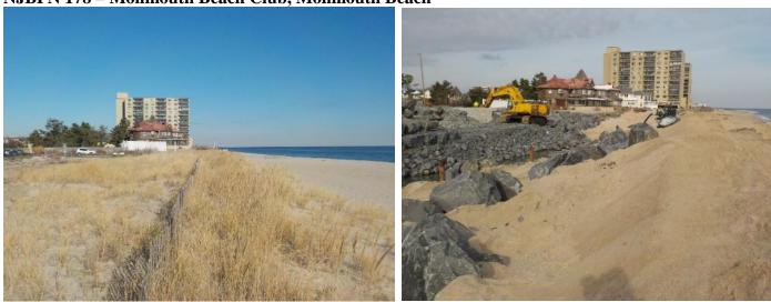
The left photo taken January 19, 2018 was taken at the sand fence line looking north across the beach berm. The right picture shows the extensive seawall construction going on at the site January 2, 2019 establishing the rock barrier to the interior.
