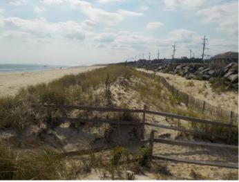
This site is near the northern limit of the initial Federal shore protection project. The left photo shows the seawall and the line of dunes looking south on Jan. 10, 2018, while the right photo (Oct. 1, 2018) shows a southerly view from the dune crest. This dune was not built as part of the project, but has developed as time passed around one line of fencing.
