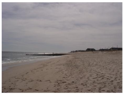
This view to the south on March 12th 2007 shows the first groin in Bay Head producing a significant offset to the south. This is common when waves move sand toward the north along this beach segment.
