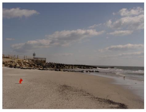
On March 5th 2007 this view toward the terminal groin shows a narrow beach with considerable exposure of the rocks. Northeast storms act to move sand around this groin where post-storm waves move it onto the beach after the storm. In the absence of northeasters sand will move up the beach from the south if southeast wave conditions prevail for extended periods of time.
