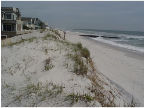
Figure 154. By the end of the summer August 28, 2007, accretion had moved substantial sand onto the berm as the offshore bar system moved close to the beach. The site gained  $23.47 \text{ yds}^3/\text{ft}$  as the shoreline advanced 26 feet. This shoreline advanced 37 feet between May 11 and August 28, 2007.
