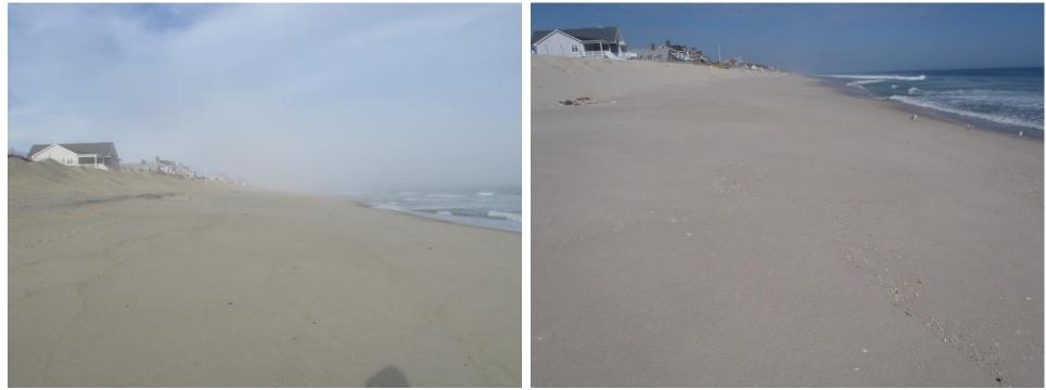
Figure 239a & 239b. The photos (left taken December 14, 2015 and right taken October 17, 2016) show the narrow dry beach that is less than 100 ft in width and sand scraped from the berm to cover the steel bulkhead which was exposed following the January 23, 2016 northeast storm. It took the borough from January to June 2016 to re-cover the exposed steel wall following that winter storm (Jonas).
