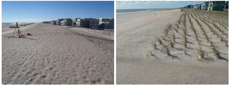
Figure 353a & 353b. The view from the dune crest at the 81<sup>st</sup> Street location shows the newly constructed dune in 2015 (left photo taken December 15, 2015) and the dune with partially planted vegetation (right photo taken October 28, 2016). Sand fencing and more planting was set to be completed shortly after the picture was taken.
