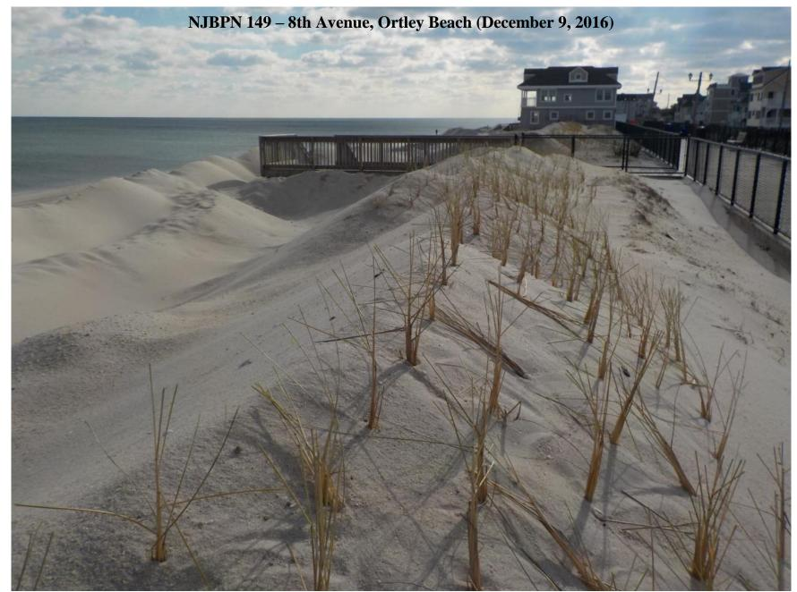
Figure 262. View to the south from the dune crest at 8th Avenue in Ortley Beach. The January 2016 northeast storm (Jonas) eroded the seaward portion of the dune. While the dune was not breached entirely, the proximity of failure was clear enough to municipal officials that they chose to add sand to the seaward dune slope for protection for the upcoming winter.
