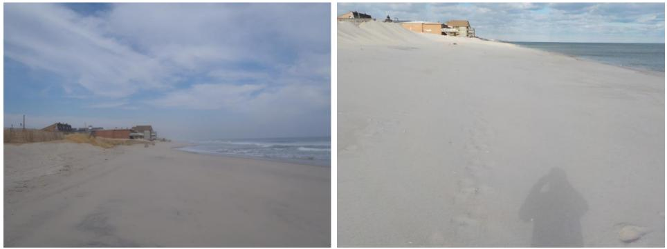
Figure 263a & 263b. The photos show the condition and width of the berm at 8<sup>th</sup> Avenue in Ortley Beach (left photo taken December 11, 2015 and right photo taken December 9, 2016). Sand was added to reinforce the dune that was damaged during the January 2016 northeast storm.
