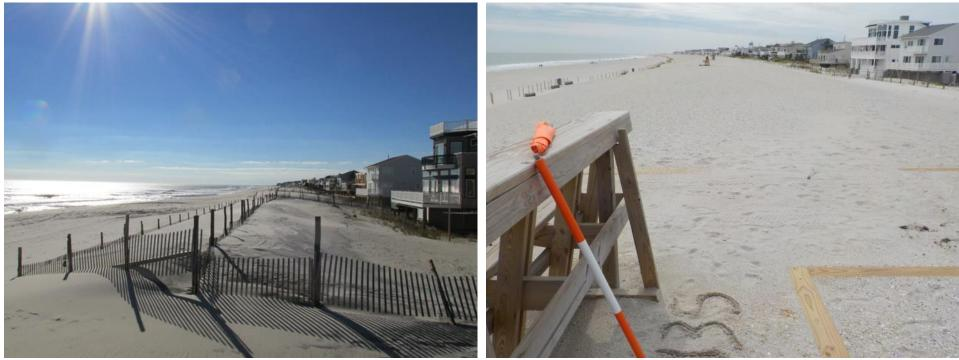
Figure 377a & 377b. The photos show the view to the south from the dune crest at Webster Avenue. The left photo (taken December 15, 2015) shows the dune that was constructed in 2013 from sand that had been recovered following Hurricane Sandy. The right photo (taken September 21, 2016) shows the condition of the engineered dune prior to fencing and planting of vegetation. The engineered dune was constructed seaward of the 2013-2015 feature.
