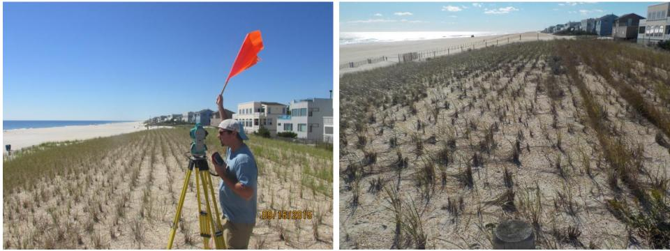
Figure 329a & 329b. Conditions of the engineered dune have remained unchanged since the completion of the post-Sandy emergency beach fill. Sand accumulated at the seaward toe during fall 2016 (left taken September 16, 2015 and right taken October 28, 2016).
