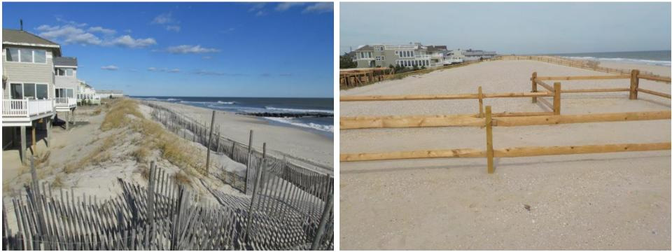
Figure 371a & 371b. The photos above (left taken December 15, 2015 and right photo taken September 21, 2016) show the drastic change in the dune at Dolphin Avenue. The narrow dune shown in the 2015 photo was created from recovered sand that was over-washed during Hurricane Sandy. The engineered dune and berm was completed during the summer of 2016.
