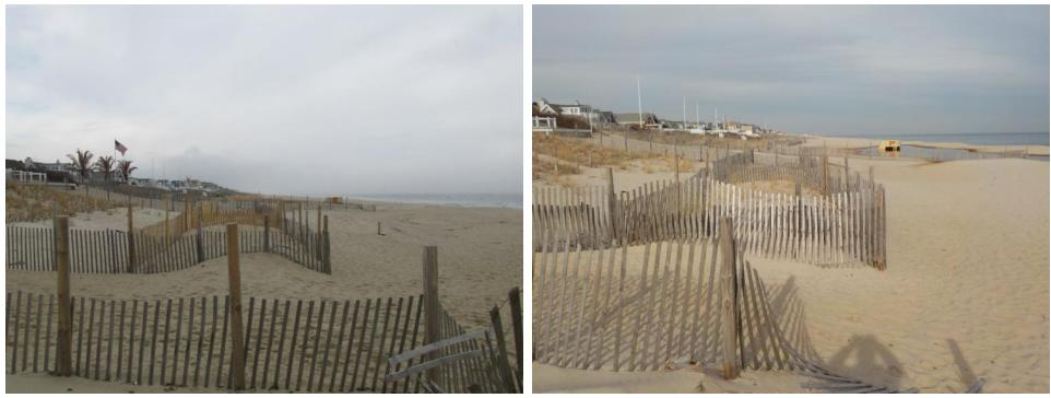
Figure 227a & 227b. The Maryland Avenue profile is located over a mile south of Manasquan Inlet. The photos (left taken December 14, 2015 and right taken December 21, 2016) show a maintained beach. Installation of sand fencing seaward of existing fence is a local effort to capture wind-blown sand. The stormwater discharge station from Sea Avenue is evident on the right photograph, but not so visible on the left.
