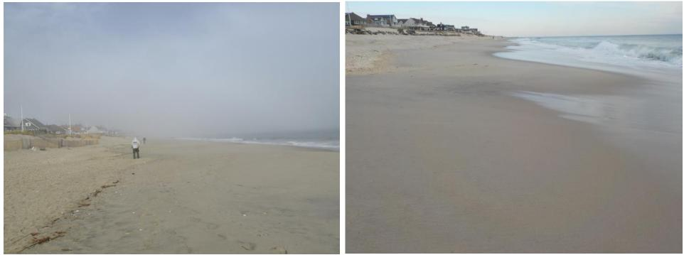
Figure 233a & 233b. Both photos (left taken December 14, 2015 and right taken December 22, 2016) show the condition of the berm at the Bay Head location. The revetment rocks were covered just prior to Jonas on the left, but were exposed on the right 11 months later.
