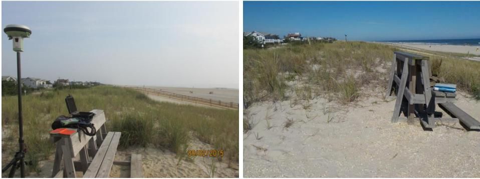
Figure 347a & 347b. The photos at 32<sup>nd</sup> Street show a stable engineered dune that has remained in place since it was constructed in spring 2012 (left taken September 2, 2015 and right taken September 23, 2016). The 2015 emergency beach fill restored the berm to the template design.
