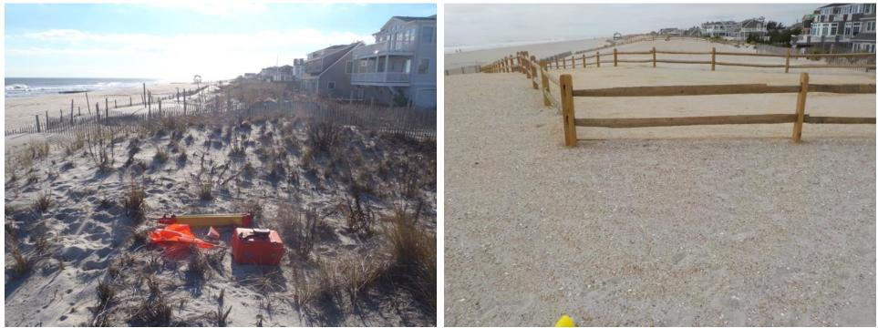
Figure 365a & 365b. The photos from the Taylor Avenue location were taken from the dune crest (left taken December 15, 2015 and right taken September 23, 2016). The engineered dune was completed at this location in spring 2016 but not yet planted by the time of the fall survey.
