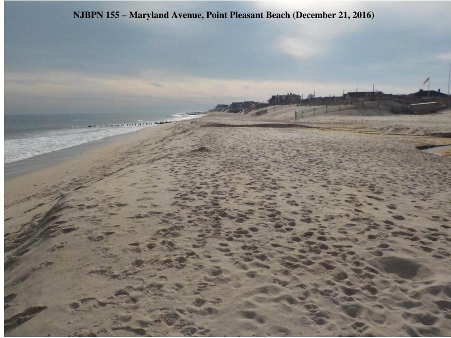
Figure 226. View to the south from the top of the berm at Maryland Avenue in Point Pleasant Beach showing the restored dune and timber groin structure on the beach
