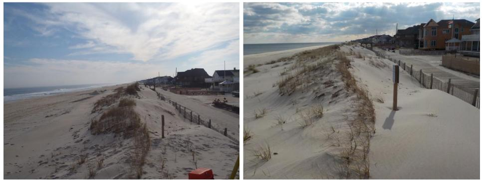
Figure 257a & 257b. The photos show the condition of the dunes at the Lavallette site (left photo taken December 11, 2015 and right photo taken December 9, 2016). Hurricane Sandy eroded the dunes at this site and these modest dunes were created from sand that was recovered after the storm. Some sand accumulated at the seaward base of the dune after the June 2015 survey.
