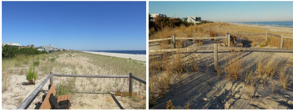
Figure 323a & 323b. The photos show the condition of the vegetation on the engineered dune that was created in the 2009 federal shore protection project. Though scarped by Hurricane Sandy's waves, the dune (and wide beach) provided the necessary protection to landward properties during the storm. The 2013 emergency fill restored the dune and berm to the original design template. Left photo was taken September 15, 2015 and right photo taken November 18, 2016.
