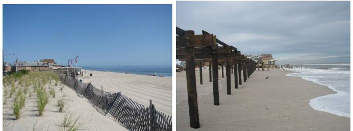
The photograph on the left (September 14, 2012) shows a modest berm and the municipal dune present prior to the storm. On the right (November 8, 2012), 68.7 yds<sup>3</sup>/ft of berm and dune were removed during the storm. Over 10 feet of dune height was pushed landward in overwash deposits. The boardwalk was located landward of the dunes (left) Ocean Avenue was destroyed as well as several homes. The photo on the right shows a classic flat beach created by the large waves.
