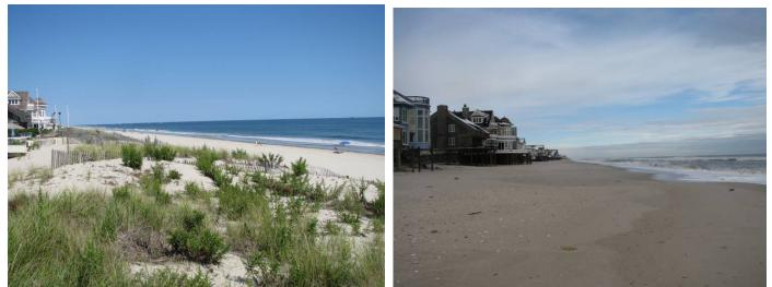
The photograph on the left (September 14, 2012) shows the limited dune system and minimal berm prior to Sandy. On the right (November 8, 2012), the photo shows damages to structures and exposure of once-buried bulkheads following the storm. Significant overwash occurred at this site and many oceanfront and landward homes were damaged.
