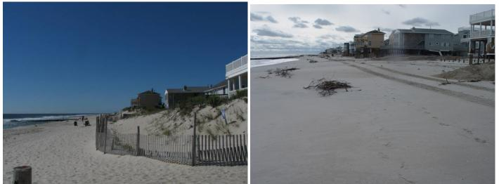
The photographs above were taken on September 10<sup>th</sup>, 2012 (left) and November 1<sup>st</sup>, 2012 (right). Both images show the view of 81<sup>st</sup> street (site 139) looking south. It is evident in the photographs that the existing dune was completely eroded away and overwash occurred, with waves pushing water and sand under the oceanfront homes and into the streets landward of them. The dune elevation was about 16 feet.
