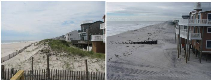
The photographs above were taken on September 6<sup>th</sup>, 2012 (left) and November 1<sup>st</sup>, 2012 (right). Both images show the view of Webster Avenue in Beach Haven (site 135) looking south. It is evident in the photographs that the existing dune was completely eroded away and overwash occurred, with waves pushing water and sand under the oceanfront homes and into the streets landward of them exposing the timber section of an old groin that was not exposed prior to the storm.
