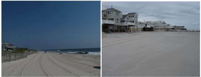
The photographs above were taken on September 6<sup>th</sup>, 2012 (left) and November 1<sup>st</sup>, 2012 (right). Both images show the view of Dolphin Avenue (site 136) looking north. It is evident in the photographs that the existing dune was completely eroded away and overwash occurred, with waves pushing water and sand under the oceanfront homes and into the streets landward of them. Damage was clear and very common.
