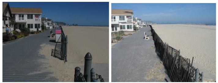
The photograph on the left was taken on September 21, 2012. The one on the right shows no noticeable change to the backbeach elevation following the storm (taken November 12, 2012). This urban beach did not have a dune system but was spared from more severe damages by the over 600-foot protective berm.
