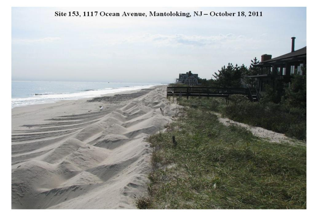
Figure 163. Shown above is the view looking south from the dune crest at 1117 Ocean Avenue in Mantoloking, NJ. Bulldozing sand from the berm to the dune slope has become a common practice in the Borough of Mantoloking.
