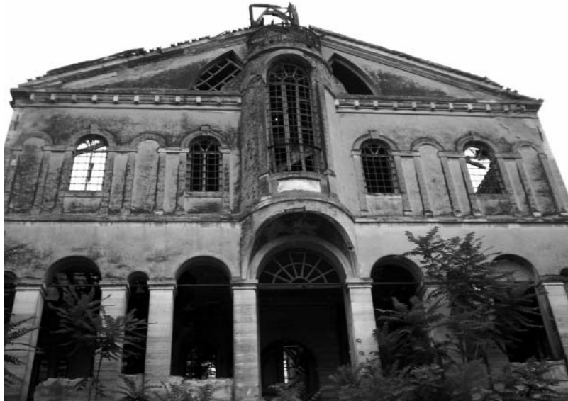
A magnificent church structure in dusty village named Dereköy near Bursa
