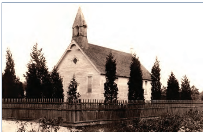
Presbyterian Church, Woodland Township, c. 1909. This lovely church was certainly built with local white cedar. Today, this edifice continues to serve the community as a Methodist Church. One of several historic photos donated to Special Collections by the Woodland Township Historical Society.
