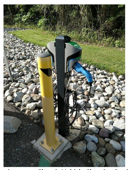
Aerovironment Electric Vehicle Charging Stations Dual Head, 208/240V @ 16A, 20' Cords
